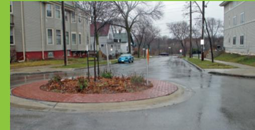
**Mini-Roundabout:** Mini-roundabouts exist at smaller, residential intersections to avoid the use of signals, or stop signs. Mini-roundabouts often consist of mountable curbs to allow for passage of large vehicles such as fire trucks and moving vans. Mini-roundabouts work in the same way as larger roundabouts in terms of right of way.
