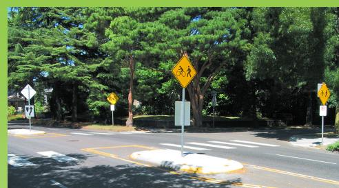
**Median Refuge:** Median refuges are raised islands in the centre of the roadway where cyclists or pedestrians can stop to wait for traffic to clear while crossing the road. This measure reduces the crossing distance, enhances pedestrian safety and allows cyclists and pedestrians to concentrate on watching traffic from one direction at a time.
