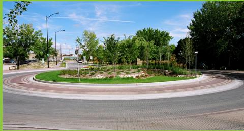
**Roundabout:** A roundabout is a form of traffic control in which traffic enters a one-way stream of traffic around a central island. Vehicles entering the roundabout yield to those vehicles already in the roundabout prior to completing left, thru or right movements thru the intersection.
